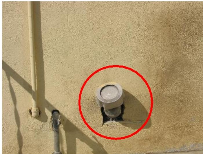
Improper installation of vent pipe. Exhaust vent from water heating in the basement area.
